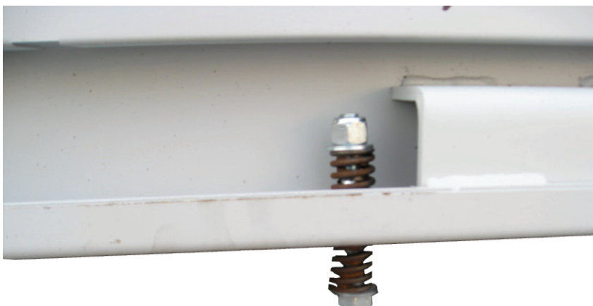
Close up of spring on flex mount floor
